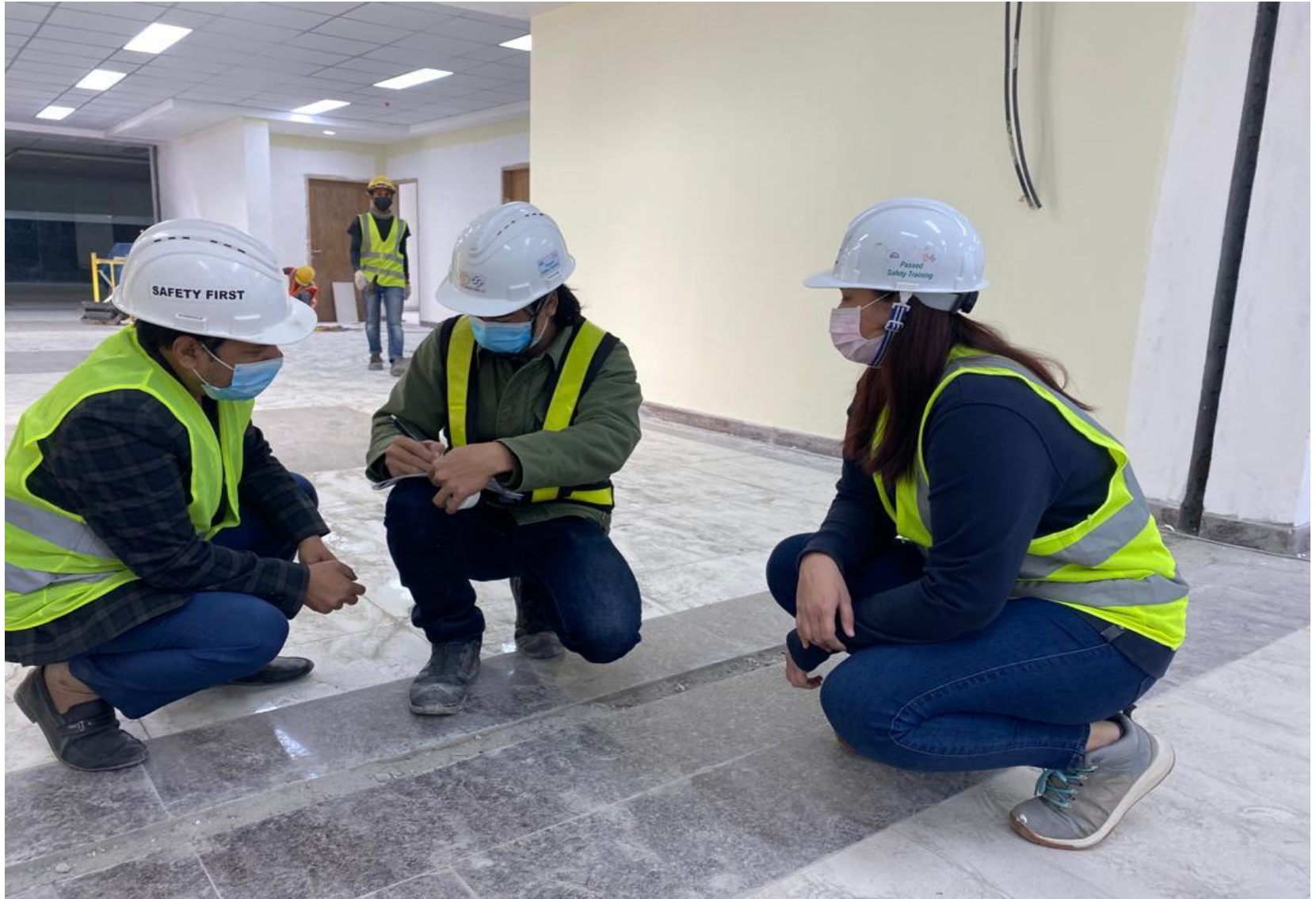
Discussion with Thai civil engineer & Architect at CP-02, Uttara
